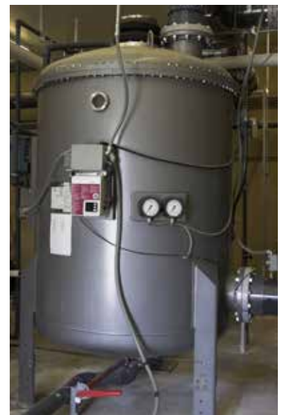
Figure 6-8 Regenerative DE Filter
